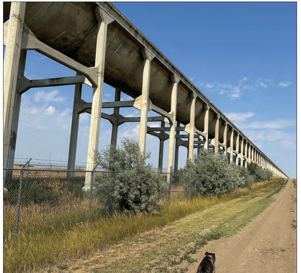
If you’re looking for a different place to walk check out the Brooks Aqueduct, a Provincial Historic Resource. The 3.2km concrete flume structure was built between 1912 and 1914 as part of the irrigation system. It sits northeast of Lake Newell and east of the city. It was the largest concrete structure of its kind in the world and is connected to the development of local farm organizations, such as the EID, which owned and operated the Aqueduct after 1935. | SANDRA M STANWAY PHOTO
