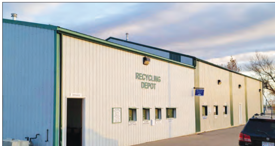
The Bassano recycling centre will be closed over the next few months. The town has been in discussions with BARRA to purchase the facility. | TOM MCPHAIL PHOTO
